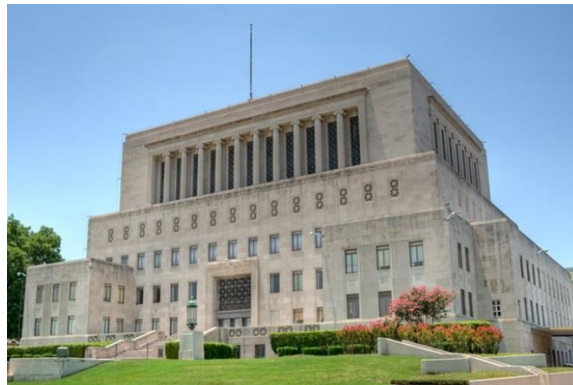
Fort Worth Masonic Temple 1100 Henderson Street, Fort Worth Texas
